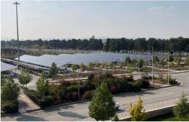
Fig. 2. Solar Photovoltaic Part of university hybrid Power Plant [8].
